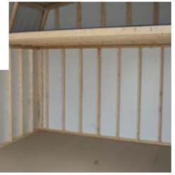
INSULATION SEEN FROM INSIDE THE STRUCTURE
